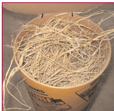
Cement form tube filled with lots of timothy or other hay. Attached to top is a cardboard circle that will cover the opening of the tube.
